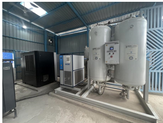
Figure 1: Conventional PSA plant
