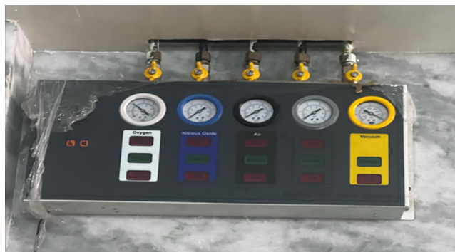
Figure 5: Area valve service unit (AVSU)
